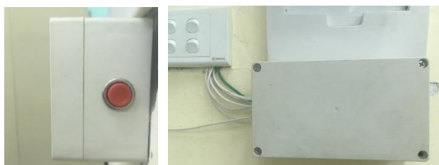
Picture 1. Device to control lamps and fans in Office
